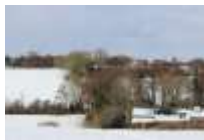
Former Waterworks 27 th February 2018
